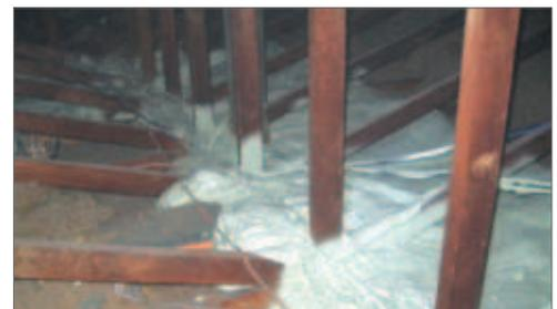
Membrane application followed by SPF application to seal off top of duct bulkhead from attic
