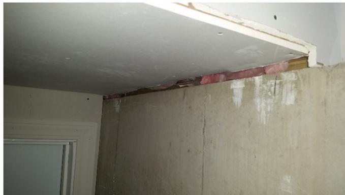
*This image is the garage side of the basement door showing the ceiling. The insulation and sill plate shown in the picture has noticeable air leaks in this area during the blower door test.*
