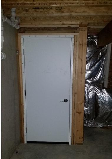
*The same door as the picture above was also not sealed around the perimeter with caulk or foam as required by code.*
