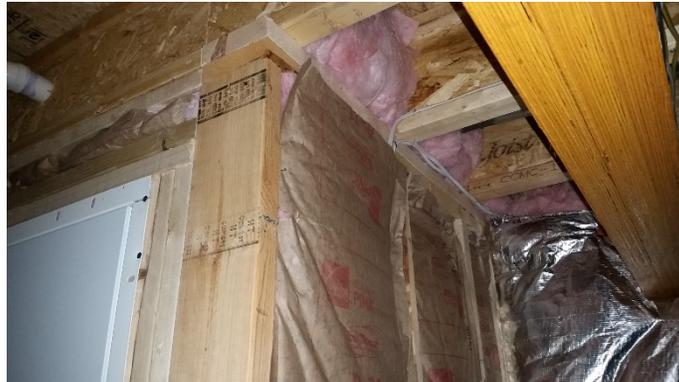
*The fiberglass insulation located in the floor joist should have an air barrier in place blocking air movement from the garage to the conditioned basement.*
