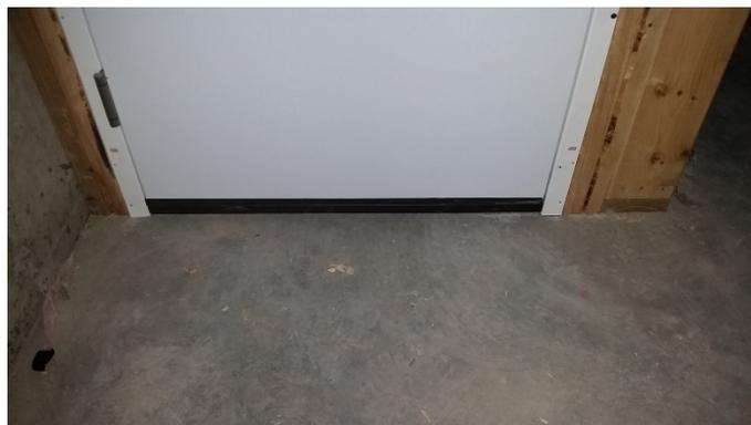
*This door installed in the basement to a stairwell leading to the garage was not sealed at the threshold. Air movement underneath the threshold indicated the door was set on the concrete floor with no caulk or gasket.*
