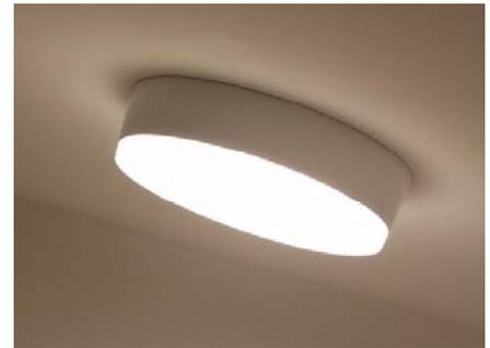
*Surface mount LEDs provide better air sealing and can help decrease leakage compared to recessed cans.*
