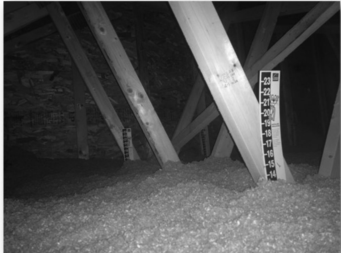
Insulation Depth Markers
